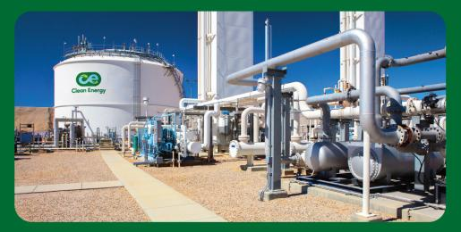
Boron, CA: 180,000 LNG gallons production per day, expandable to 270,000 LNG gallons per day. 1.8-million-gallon LNG storage tank.
